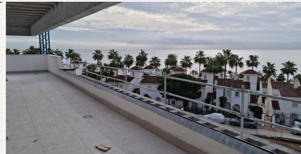
Under the roof's edge
